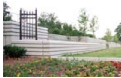
Planters were used on the north side of the bridge to hide the interstate. Photo: ARCADIS U.S. Inc.
