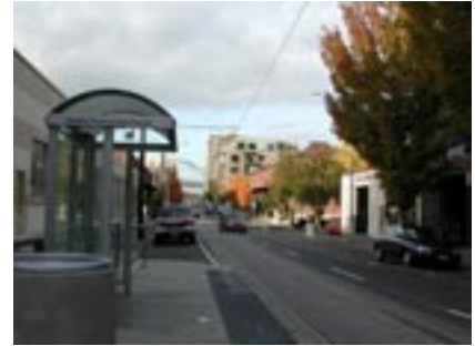
Streetcar station in Portland
