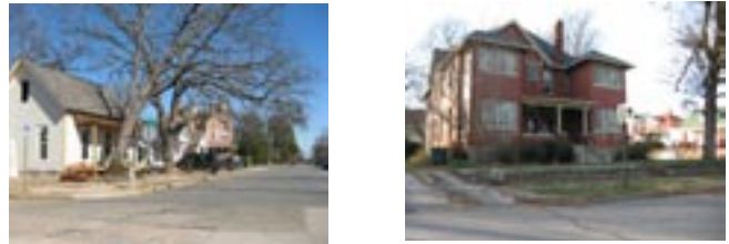
Existing and remodeled housing
