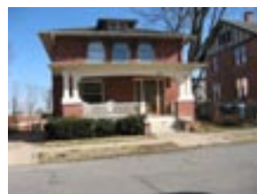
Governor's Mansion Residential - remodel
