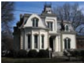
Villa Marre - restored residential
