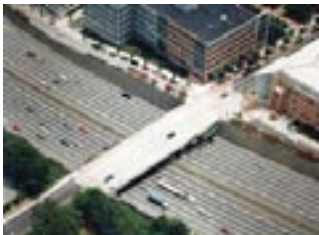
Original Fifth Street Bridge. Photo: Sunbelt Structures Inc.
