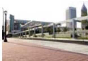
A wide sidewalk and trellis were used on the south side of the plaza. Photo: ARCADIS U.S. Inc.
