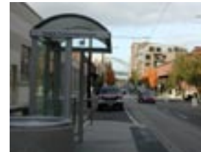
Streetcar station in Portland
