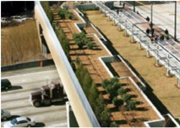
View of Atlanta Fifth St. Pedestrian Bridge
