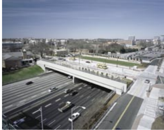
View of Atlanta Fifth St. Pedestrian Bridge
