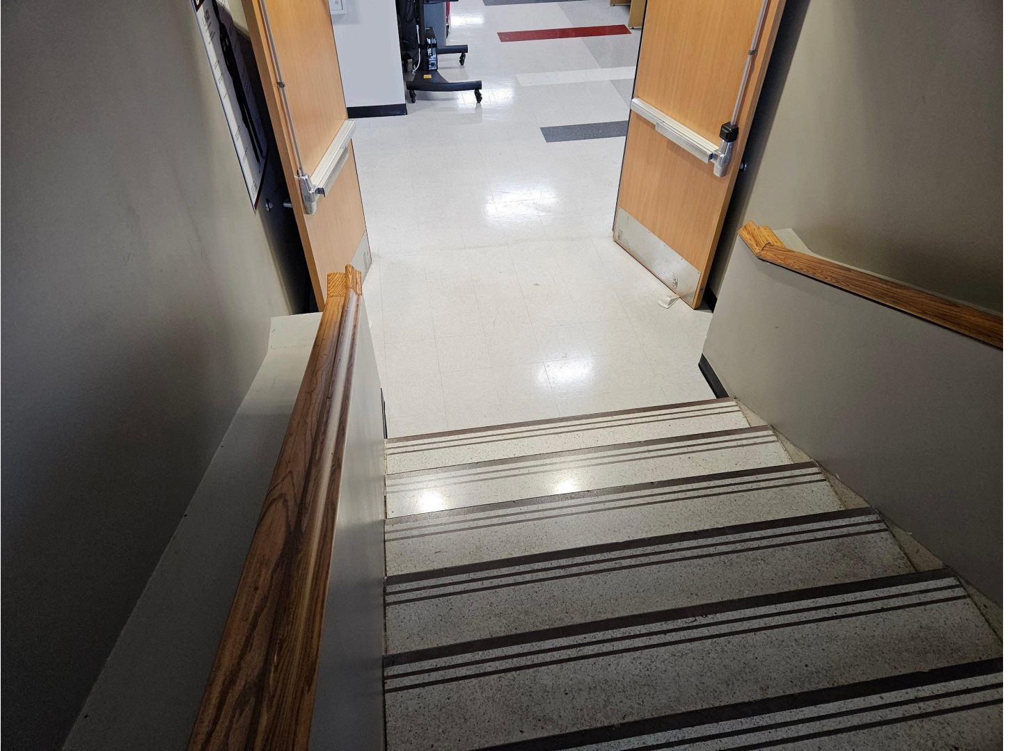
Stairwell to 1st Floor Photo 2
